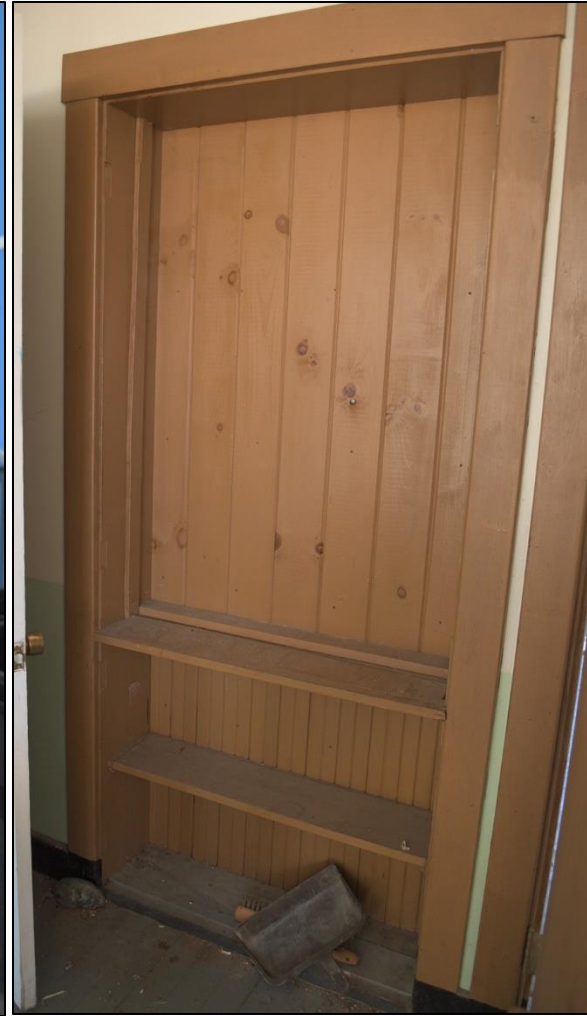
Figure 23: Built-in bookcase at east wall, entry
