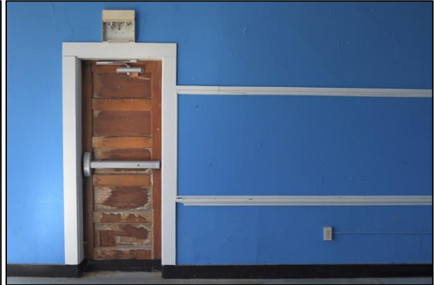
Figure 75: Egress door at north wall of north classroom
