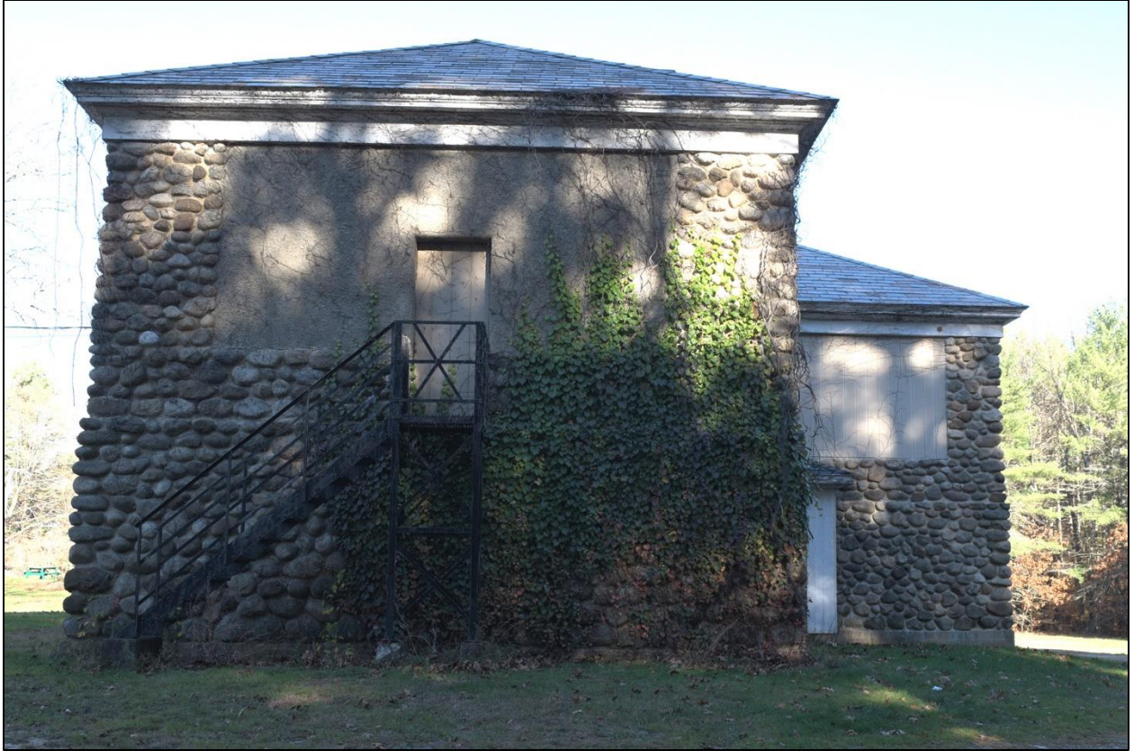
Figure 18: South elevation, Old Stone School
