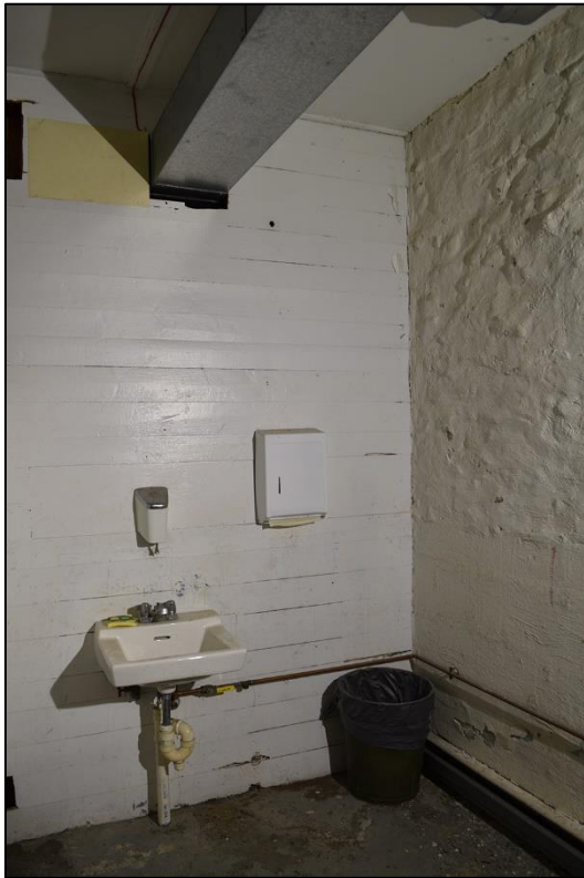
Figure 51: Sink in boys' restroom, facing northeast
