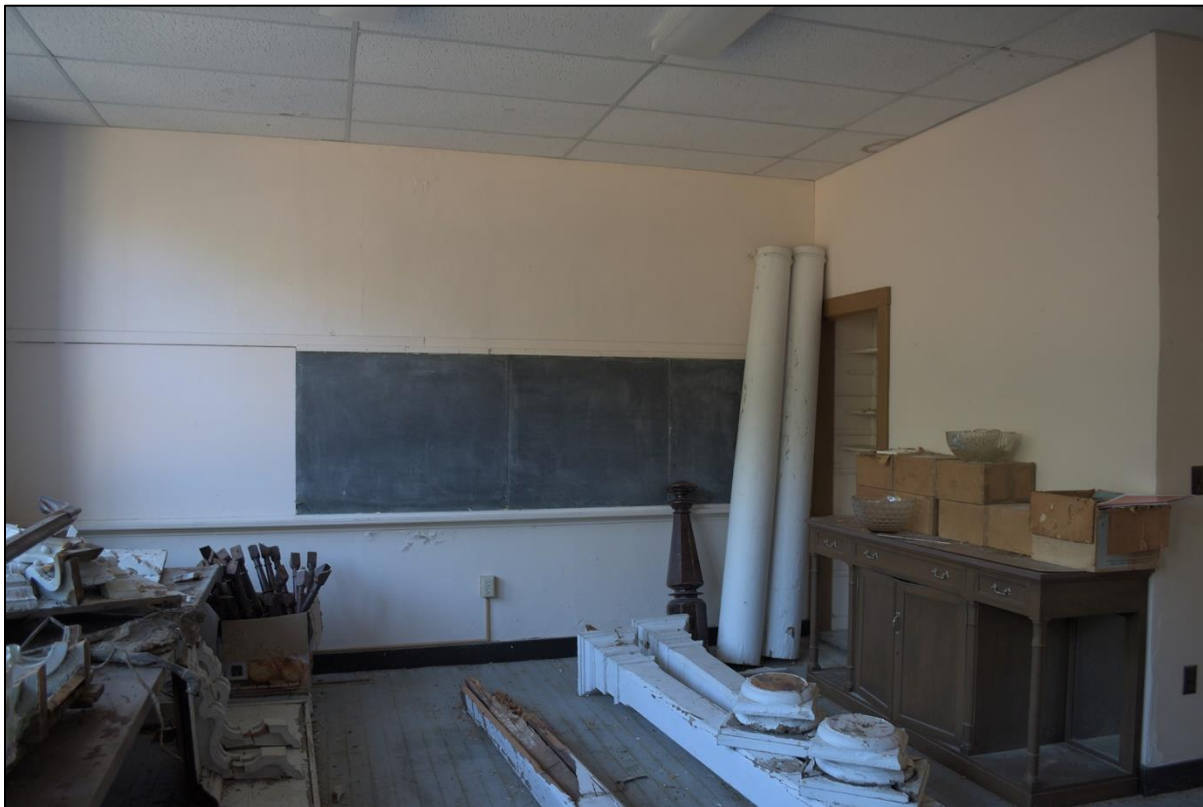
Figure 32: Ell classroom, facing southwest
