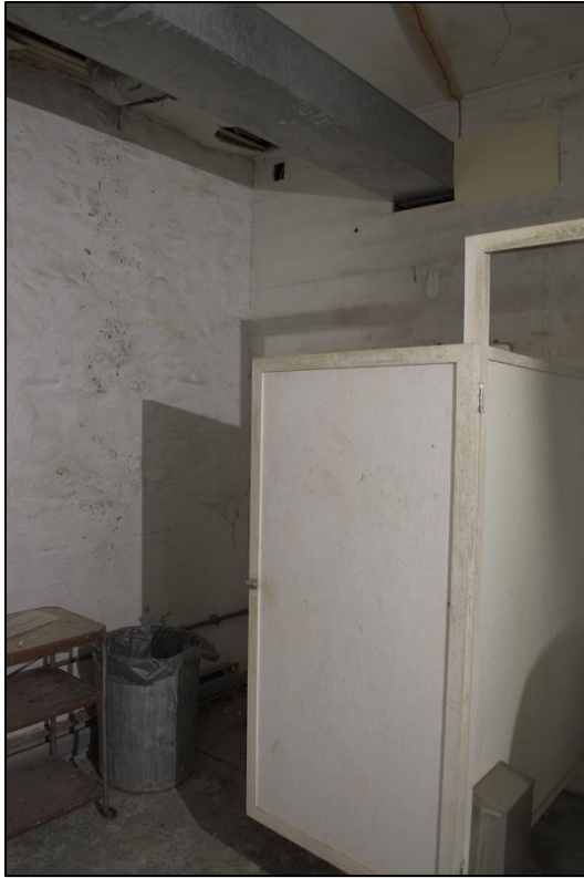
Figure 49: Girls' restroom, facing southeast
