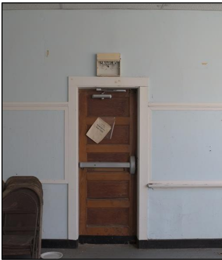
Figure 28: South fire-escape door
