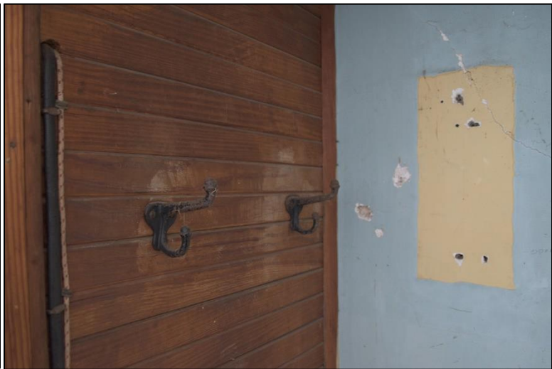
Figure 29: Horizontal beaded board and coat hooks inside of south closet
