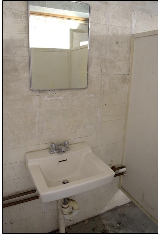
Figure 50: Sink and mirror in girls' restroom
