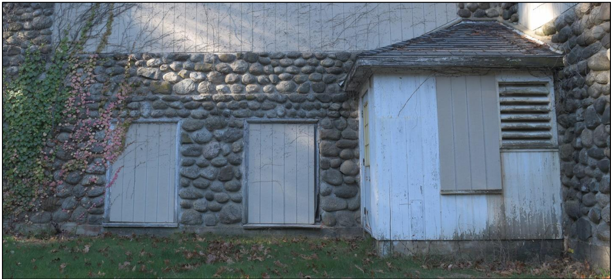
Figure 68: East elevation of south vestibule showing boarded window and louvered vent
