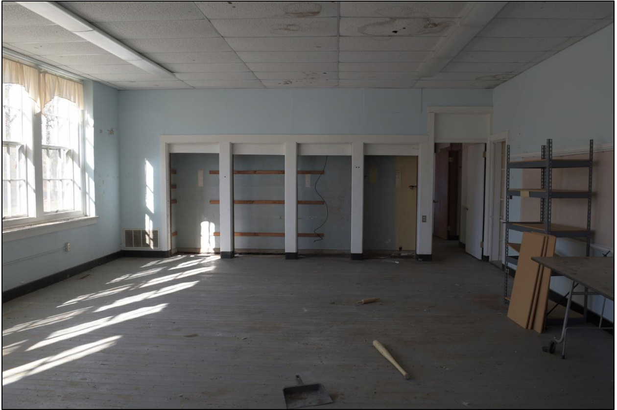
Figure 27: Interior of south classroom, facing north toward entry hall
