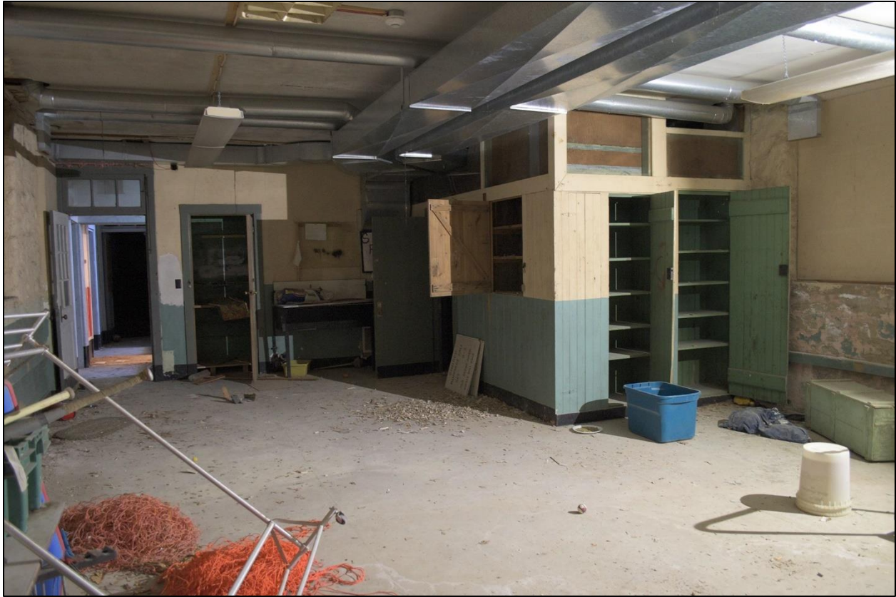
Figure 38: North storage room, facing southwest
