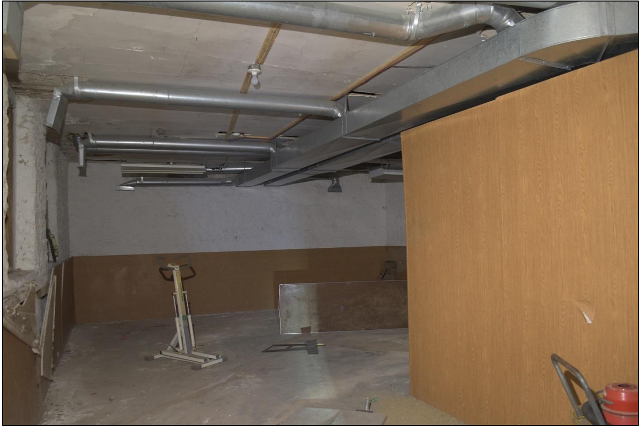
Figure 43: South storage room, facing south from entry
