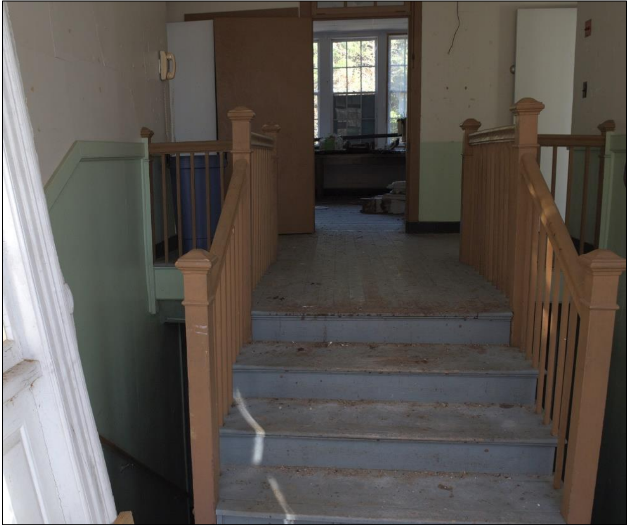
Figure 21: Entry hall, facing east, toward ell.
