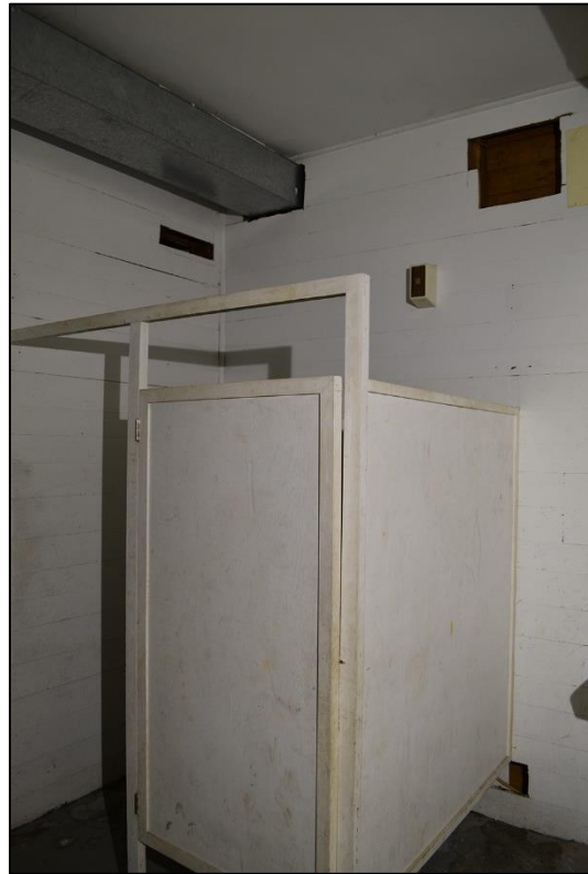
Figure 52: Stall in boys' room, facing northwest
