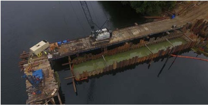
Similar Cofferdam Project
