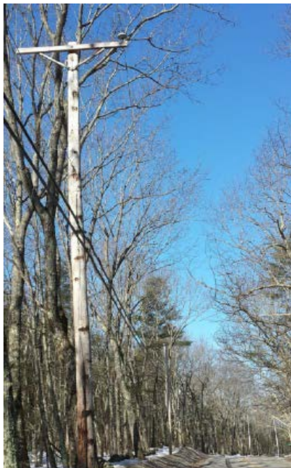
Existing Open Wire
