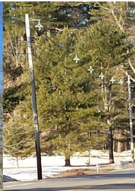
Proposed 3-phase Hendrix Spacer Cable
