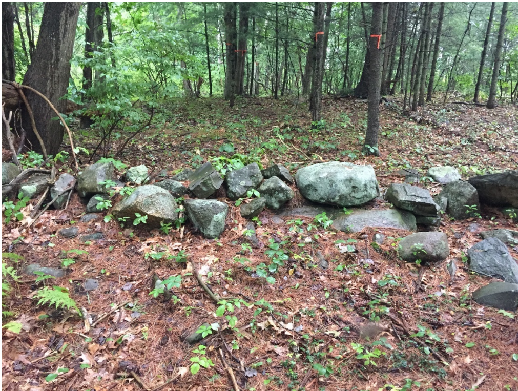
Figure 7. Stone wall WP-47, facing northwest.
