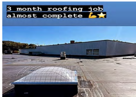
Rye Elementary School roofing / skylight work
