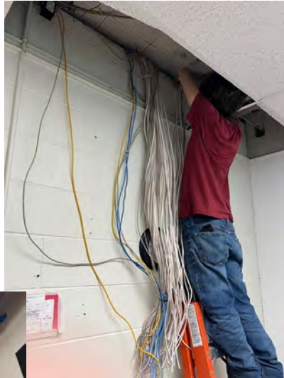
Old Wiring being pruned out
