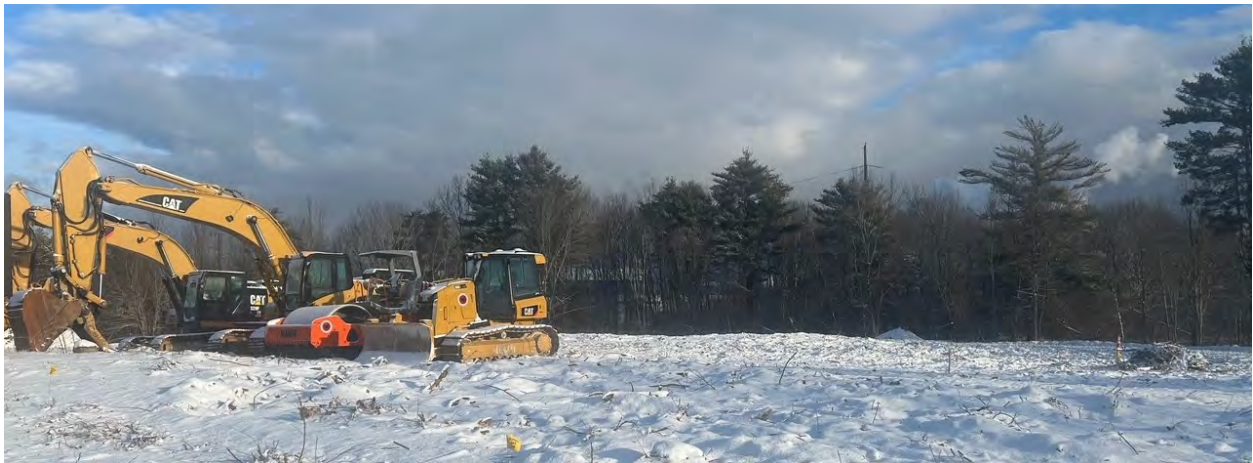
Choice Hotel site under construction- Woodbury Avenue
