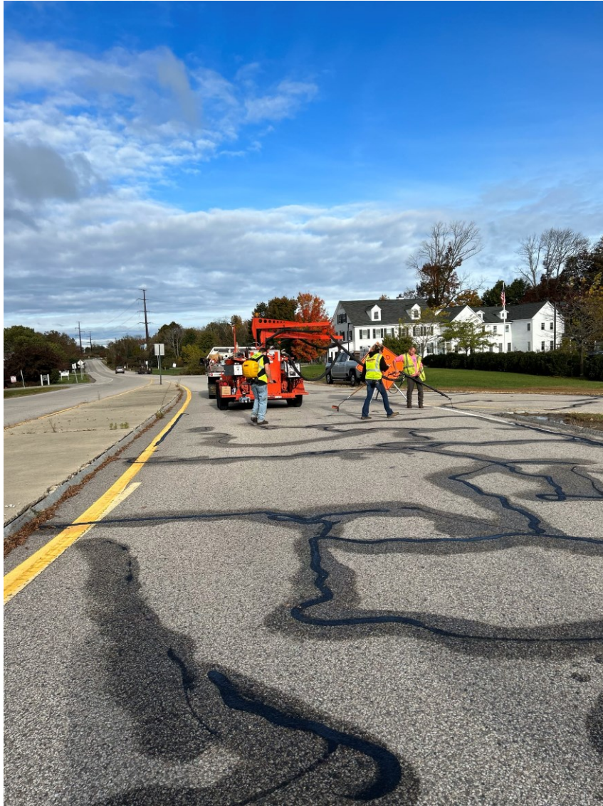
Crack sealing Shattuck Way was finished in October
