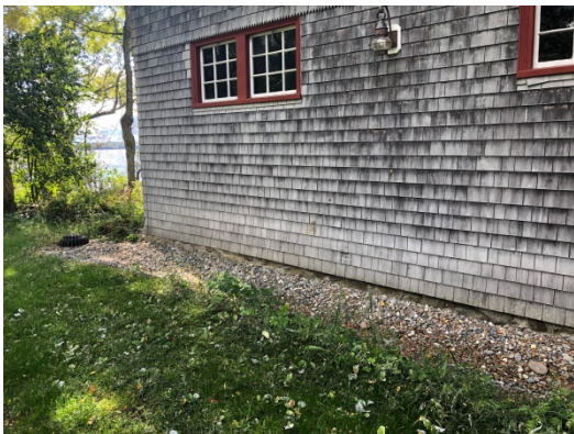
Side view with new drainage pipe installed and stone on top
