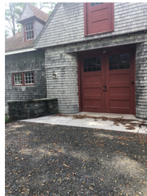
Front view with drainage installed and granite entry
