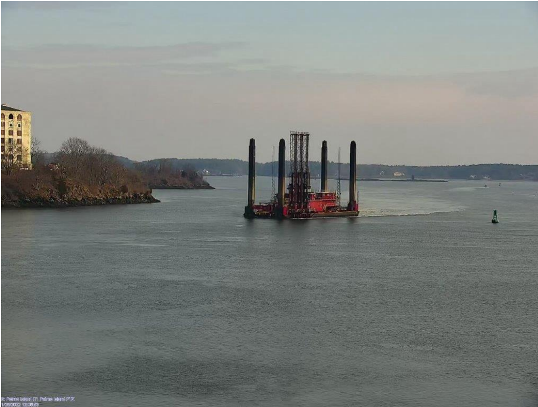
Drillboat "Apache" on its way to the Piscataqua turning basin widening project -heading to Newington
