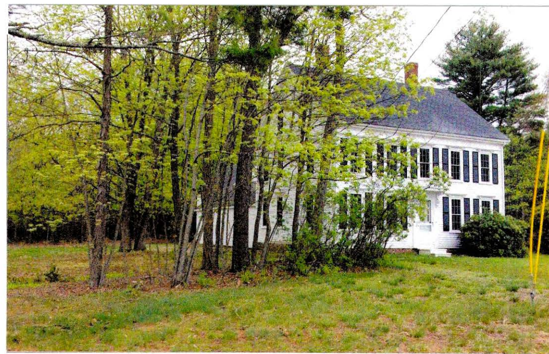
NORTH VIEW FROM NETTLE HILL ROAD
